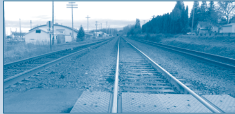
BNSF rail line looking north at Division Street crossing
